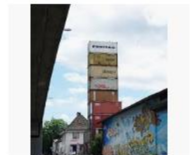
Residential Shipping Contai... residentialshippingcontainerpr...
